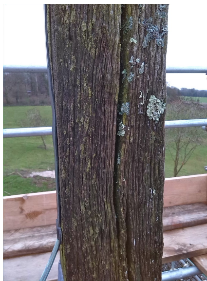
Finial crack allowing water ingress behind lead flashing
